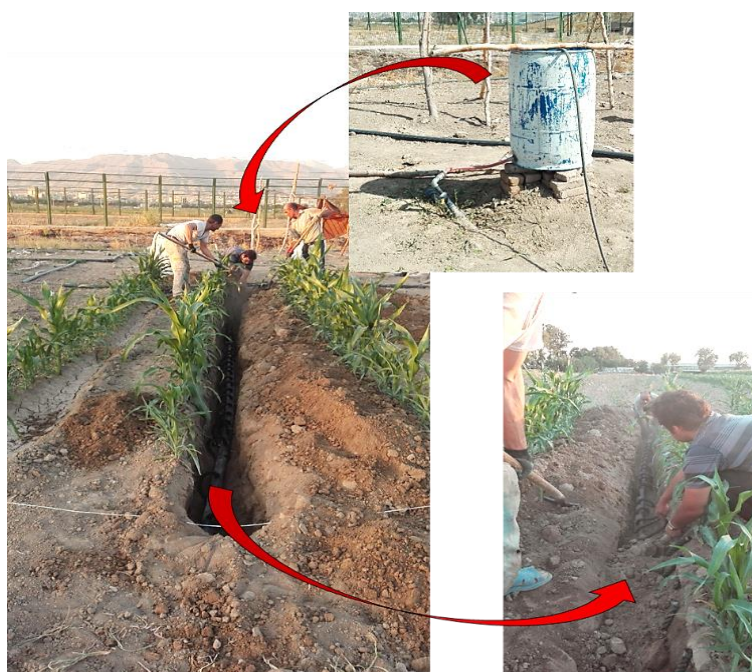
Fig. 1 Placing the pipe at a depth of 0.5 m and connecting to water reservoir and setting the wicks vertically next to the roots of the plants and filling the furrow
